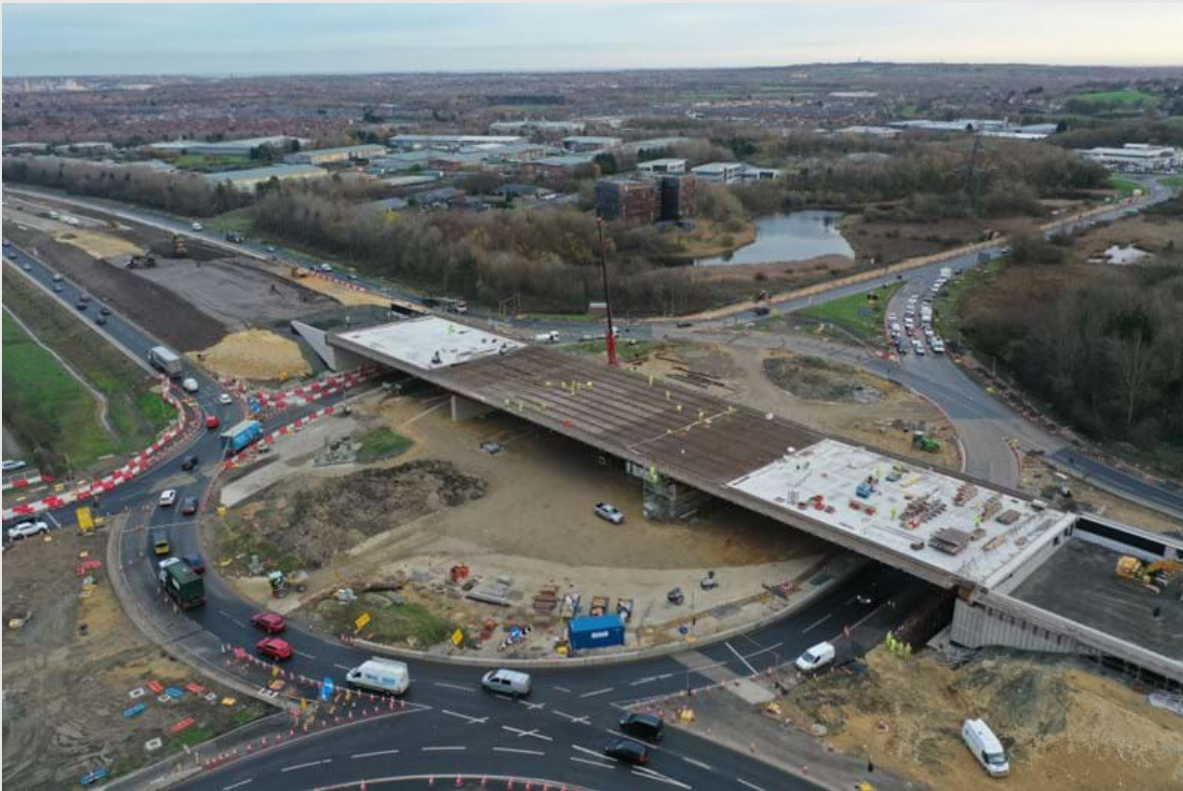
Image 6 – Junction construction works (Courtesy of National Highways)
