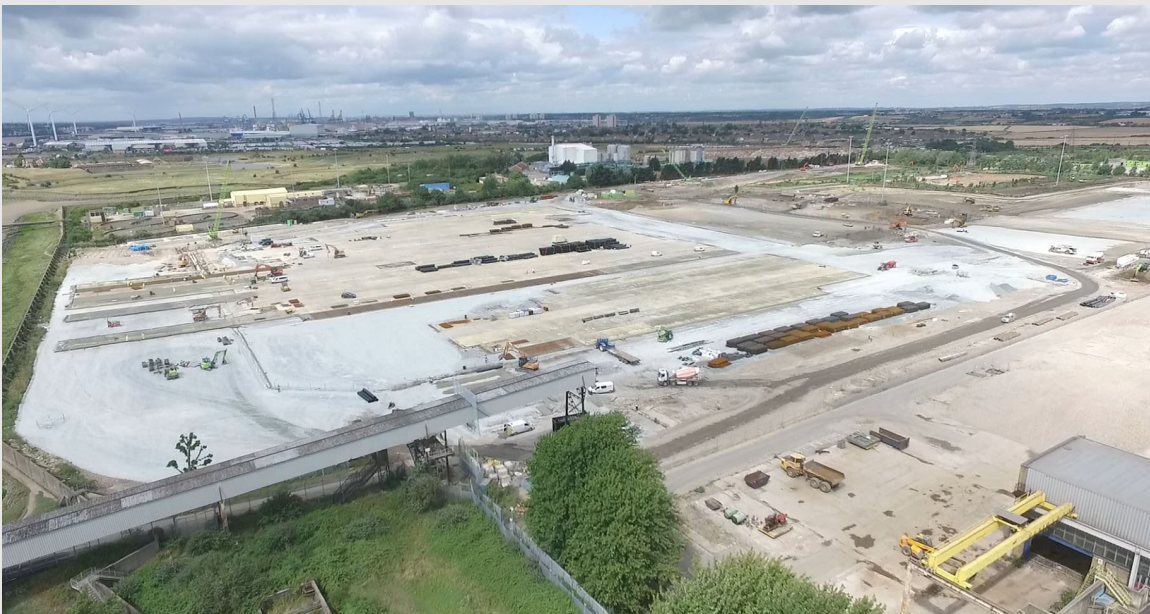
Image 5 – Tilbury2 in construction (Courtesy of Tilbury Port)
