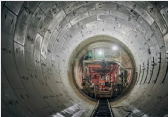
Image 3 - Thames Tideway Tunnel: Secondary lining the main Super Sewer tunnel beneath Blackfriars Bridge (Courtesy of Tideway)
