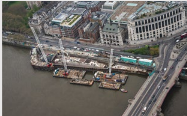
Image 4 - Blackfriars Bridge Foreshore showing surrounding cofferdam (Courtesy of Tideway)
