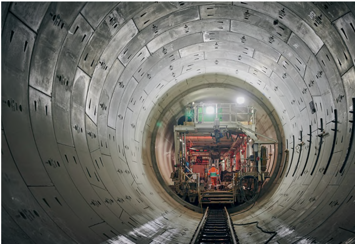
Image 3: Thames Tideway Tunnel: Secondary lining the main Super Sewer tunnel beneath Blackfriars Bridge (Courtesy of Tideway)
