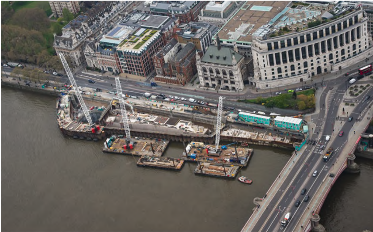
Image 4: Blackfriars Bridge Foreshore showing surrounding cofferdam (Courtesy of Tideway)
