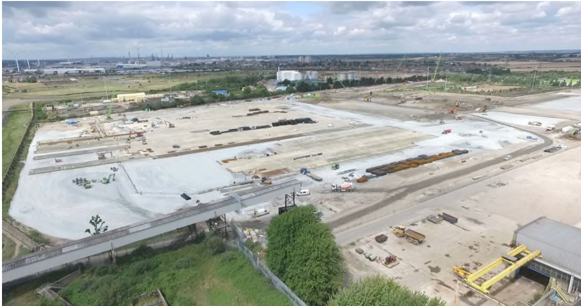
Image 5 – Tilbury2 in construction (Courtesy of Tilbury Port)
