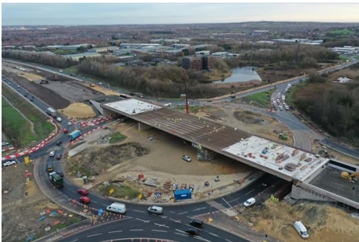
Image 6 – Junction construction works (Courtesy of National Highways)
