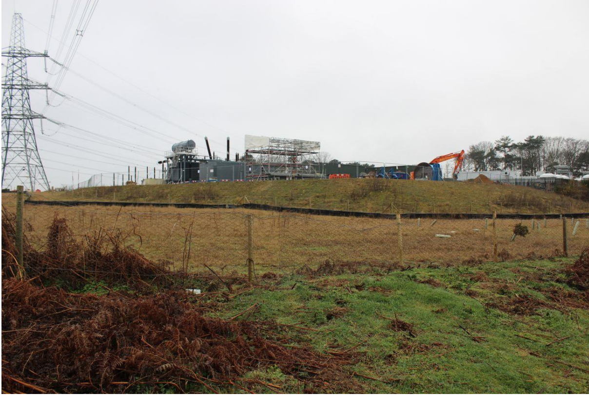
Figure 19: Construction works for the Galloper sub-station, Sizewell. (Source: Ben Clifford, 2017)
