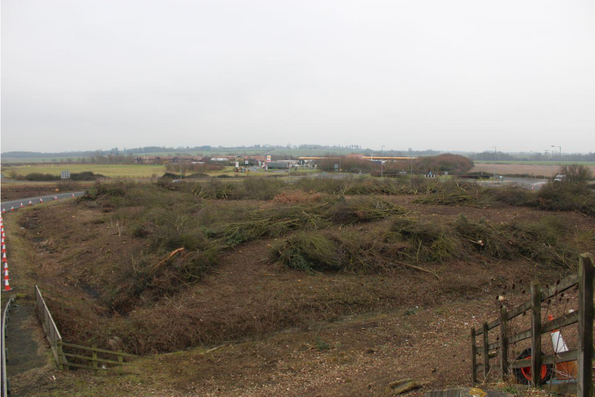
Figure 7: Site clearance near Cambridge services. (Source: Ben Clifford, 2017)
