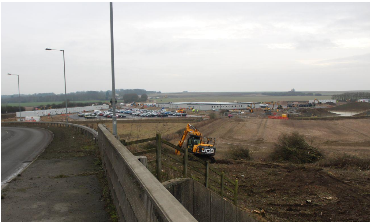
Figure 6: A14 construction compound near Cambridge Services. (Source: Ben Clifford, 2017)
